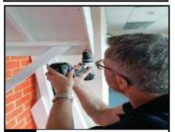
Insert 2 screws through front edge of gallows bracket into the front canopy profile
