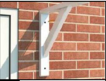
Hold a gallows bracket against the wall, at the required height, (normally just above the top of the door frame) so that the inner edge is on the line drawn.
