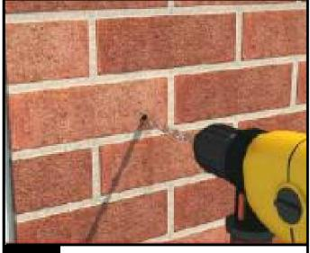
3 Mark the bottom gallows bracket hole postion
